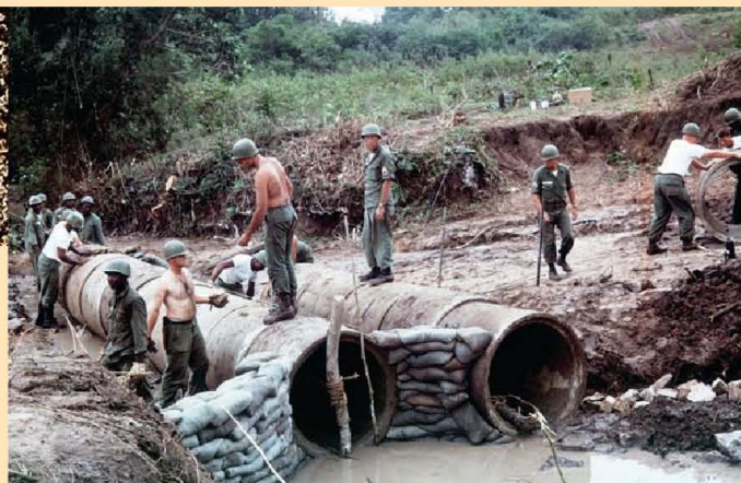
Members of the 70th Combat Engineer Battalion work on a road culvert in 1965. The unit earned a Presidential Unit Citation.
