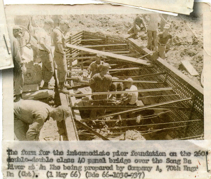
The construction of a 260' double-double, class 40, panel bridge over the Song Ba River at An Khe by Company A, 70th Engr Bn (Cbt). (9 May 66) (Bde 66-1030-937)
