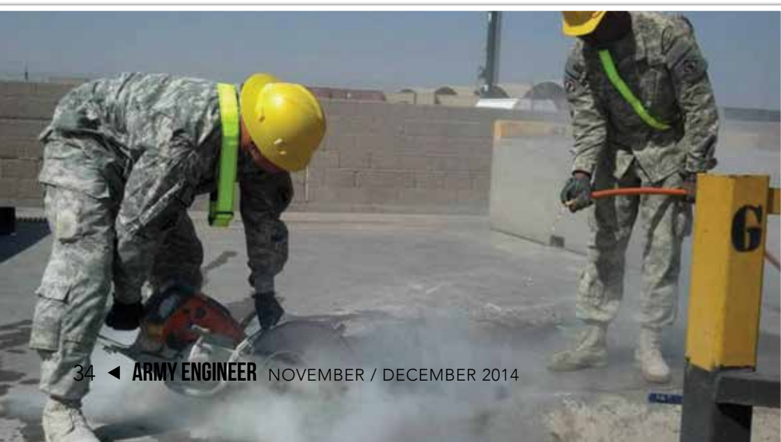
◀ In support of construction operations at Camp Arifjan, a soldier from the 76th EN Co. operates a concrete grinder while a fellow soldier waits with a hose to cool down the blade. PHOTO BY 1LT MICHAEL CADDIGAN
