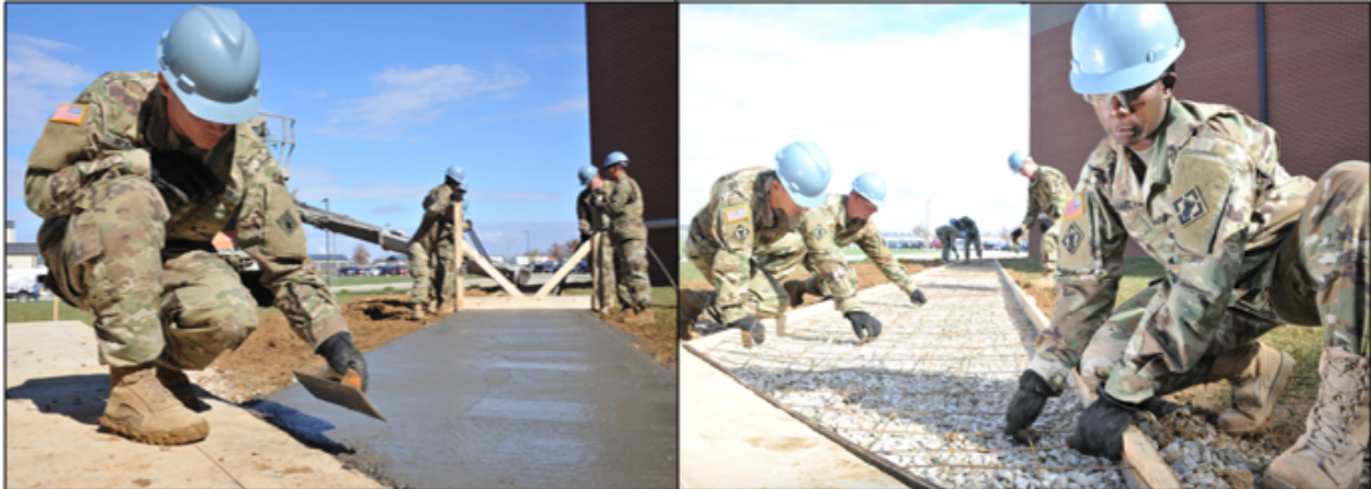
The 76 th EN CO (V) places a concrete sidewalk at the Battalion Barracks in order to allow Soldiers and families to access the recreational area.
